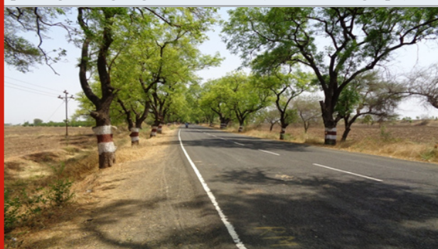
Figure 2: State Highway from Amravati to Paratwada passing through agricultural land (Actual Photograph)
