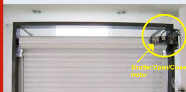
Figure 3: Shutter with motor operated
