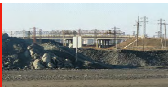
Fig. 2: The overpass of the industrial site of the open-cast in the Maykain mining affected area
