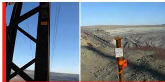
Fig. 4: The deformation control benchmarks were installed in September, 2011 on the ETL supports and caving coil in the monitoring station No 1 area
