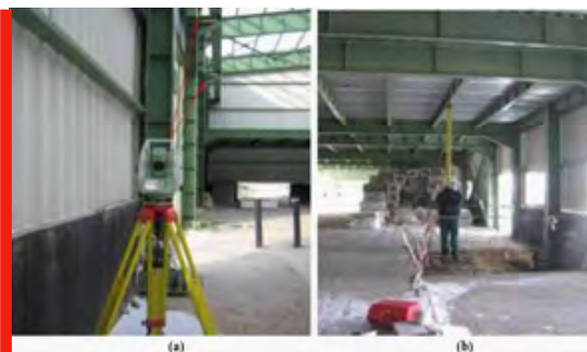
Fig. 5: a- determination of the deformations of the ETL substation b- determination of the beams sag of the PP building covering
