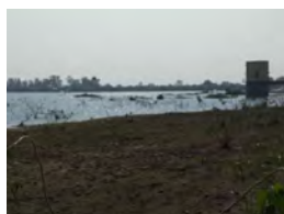
Borala Dam (Adol Dam)
